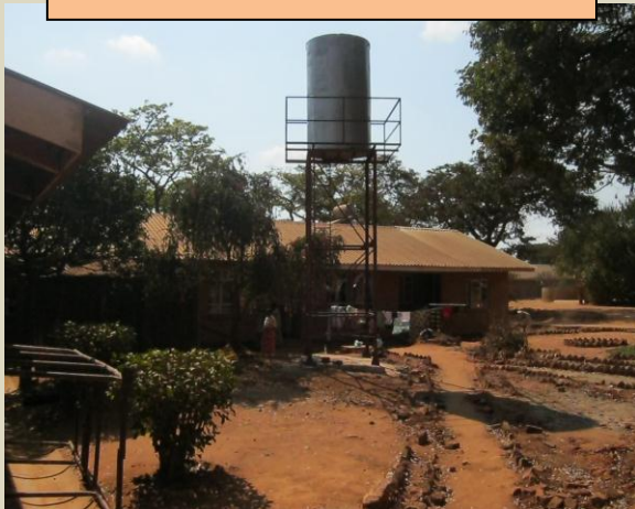
The new water tank, adjacent to the maternity ward.
